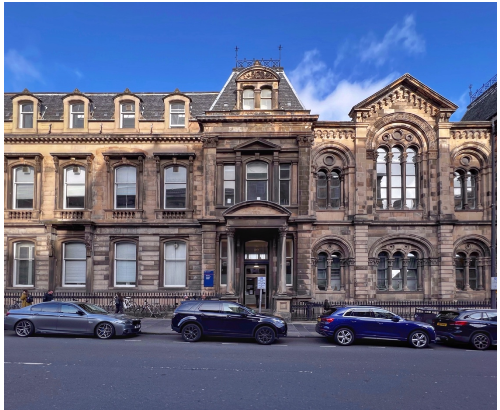
Figure 7. Edinburgh School of Architecture and Landscape Architecture. Photo: Author, from Churchill Fellowship.
